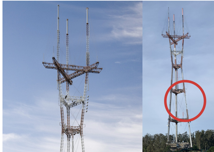
A photo-simulation of the top of the tower with the new "repack" antennas and open truss legs, and the 90-foot open truss test section as viewed from Twin Peaks
