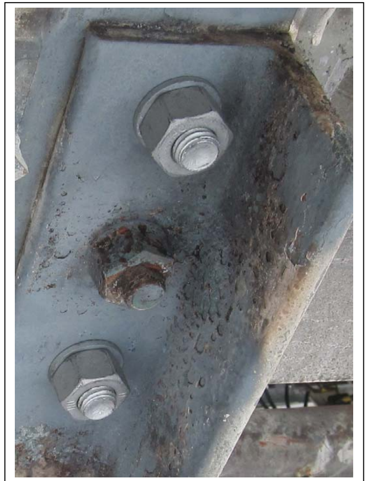
Photo No. 22 (After)
