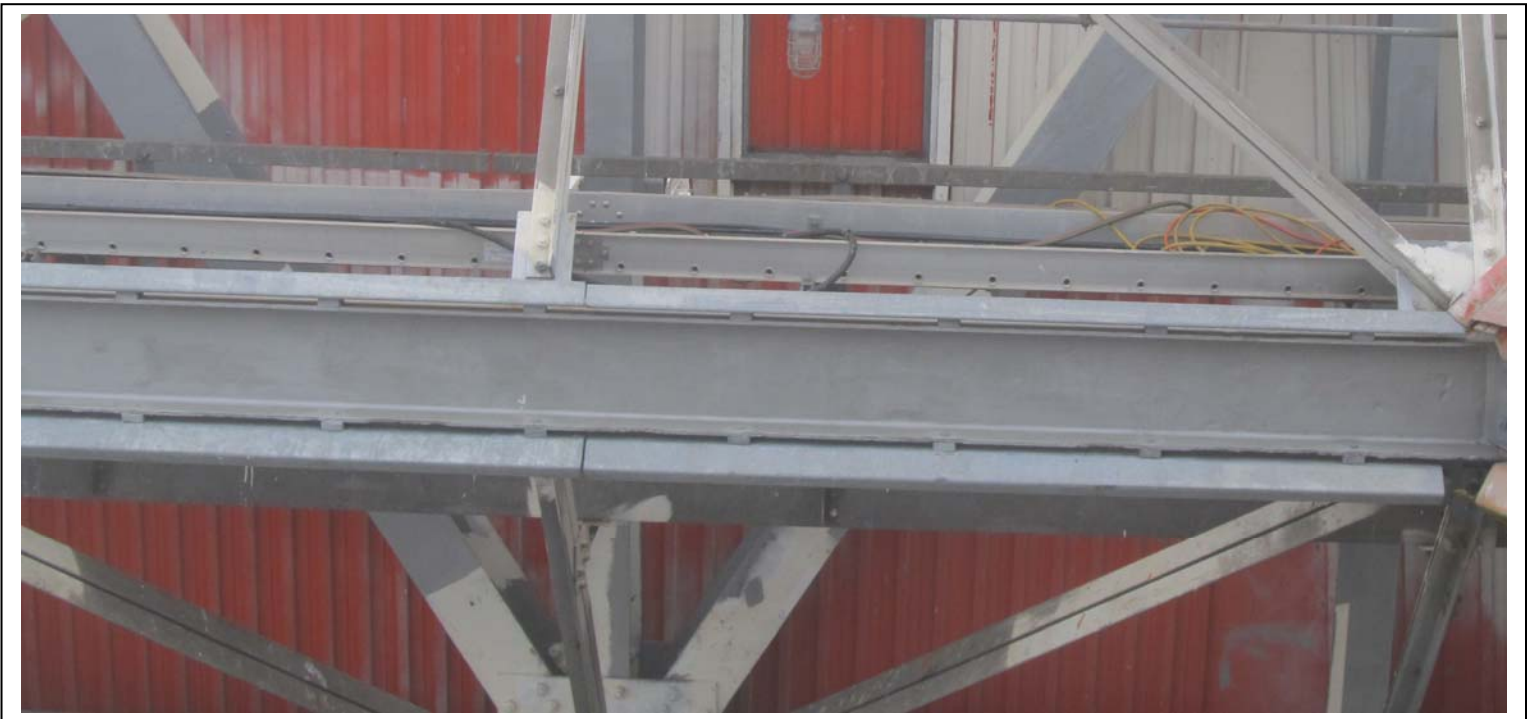
Photo No. 5 (After)
