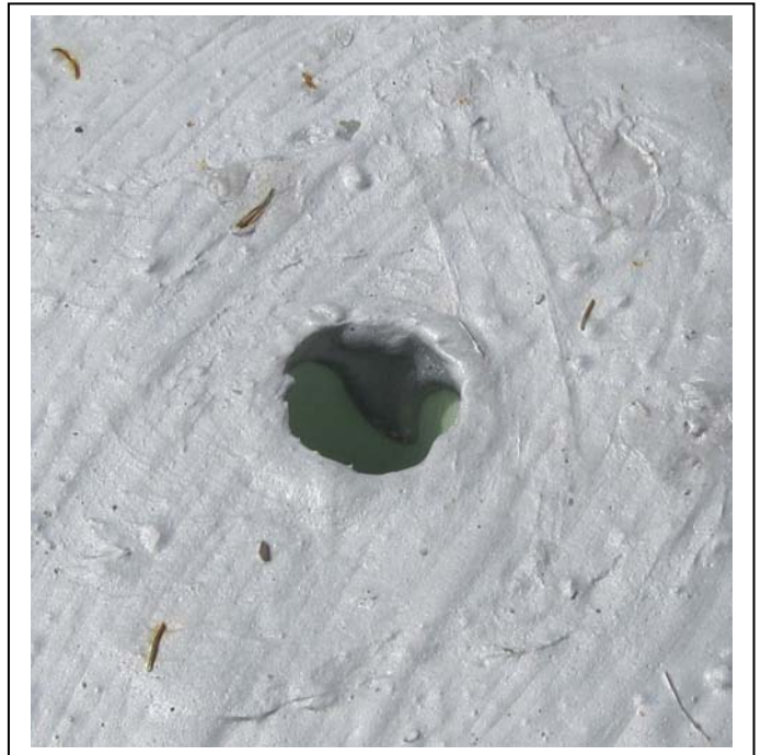
Photo No. 33 (After)
