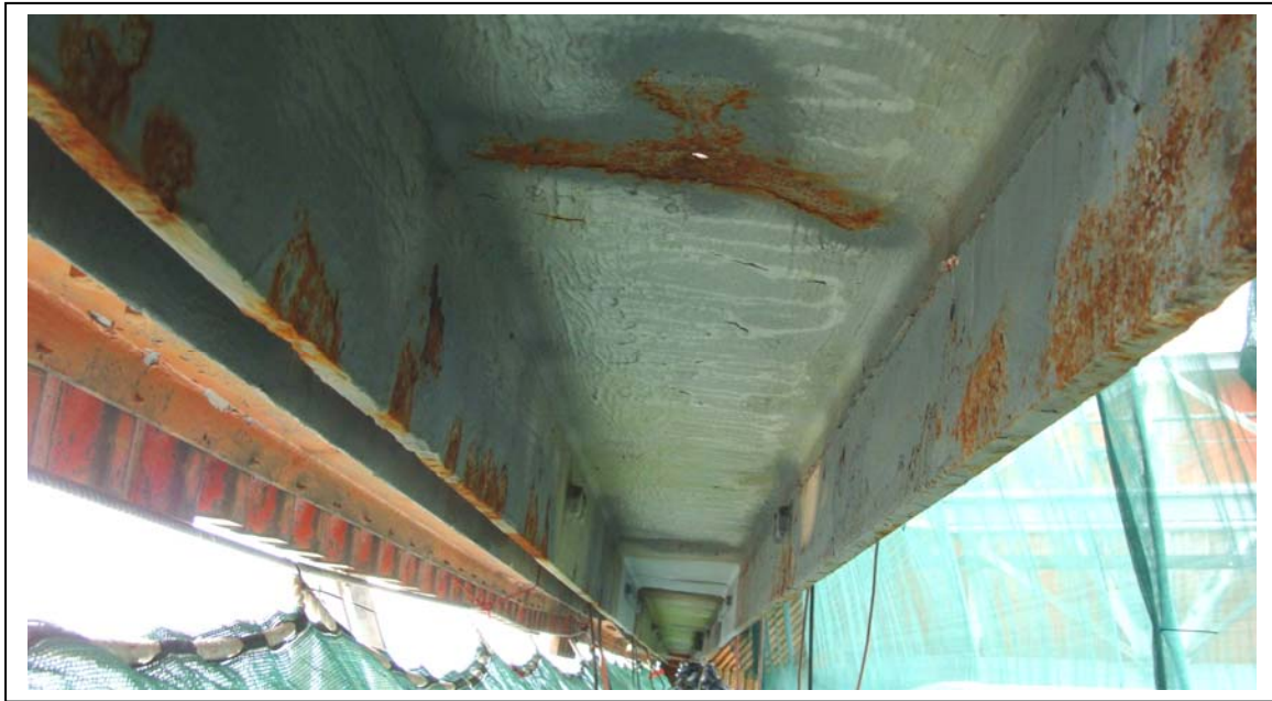
Photo No. 12 (Before)
