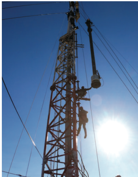
Tower workers removing the old KGO-TV antenna
