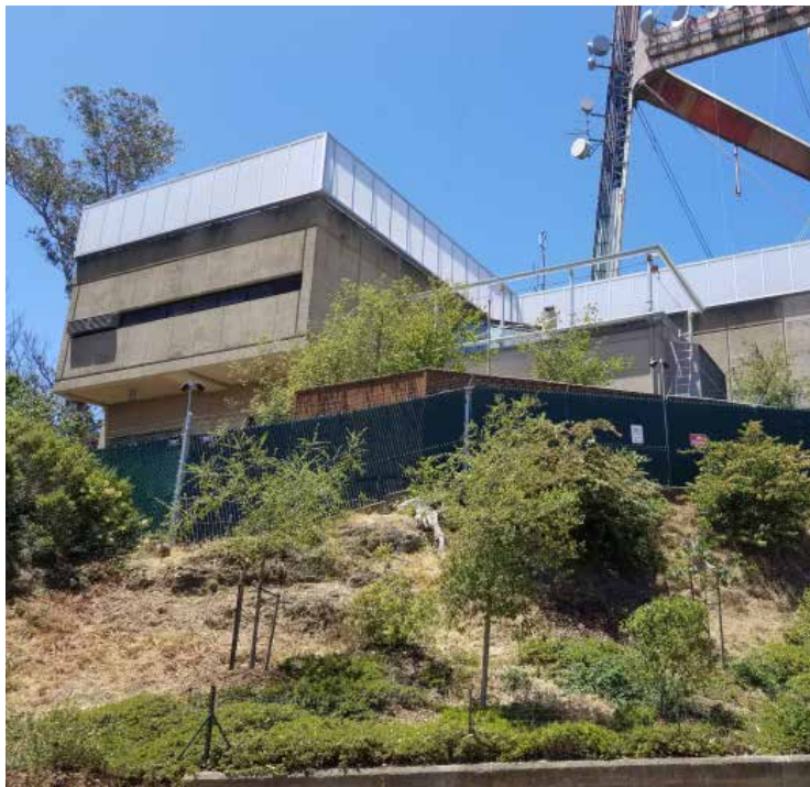
Native plants on the hillside and parapets on the building enhance the view from the reservoir trail
