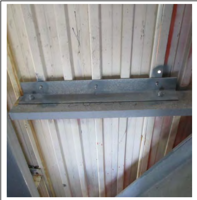
Photo No. 16 (After)
