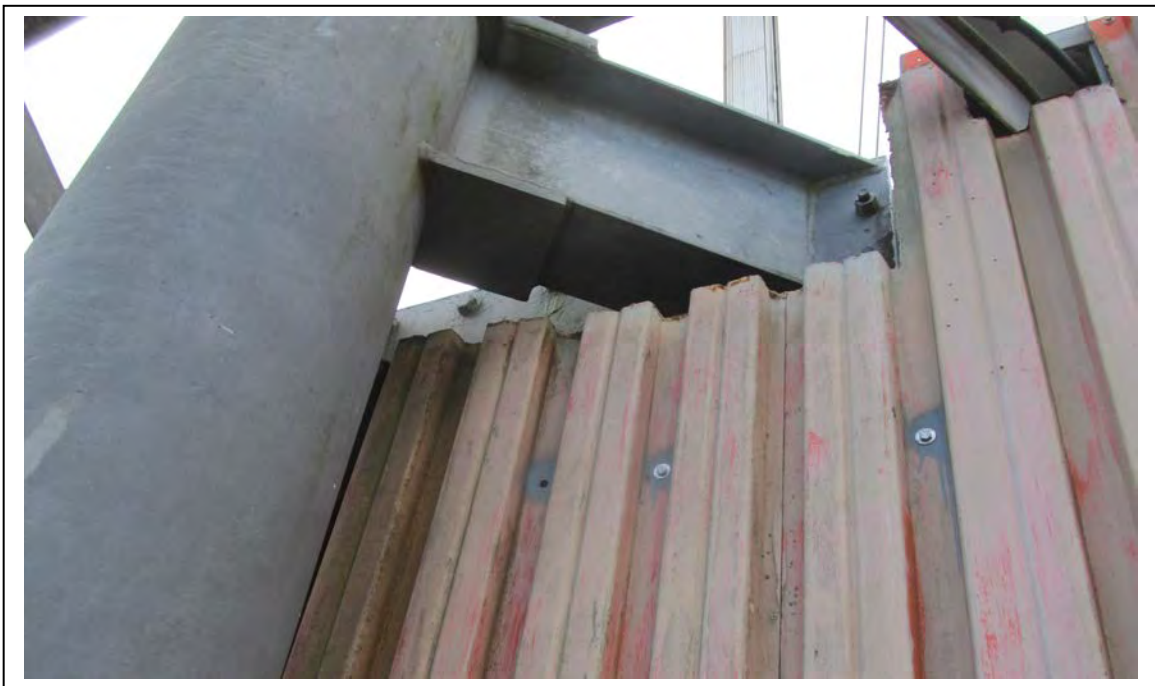
Photo No. 12 (After)
