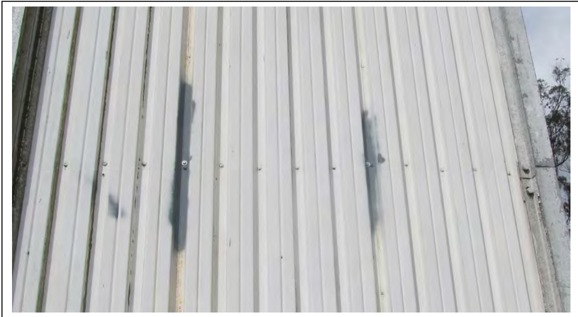
Photo No. 15 (After)
