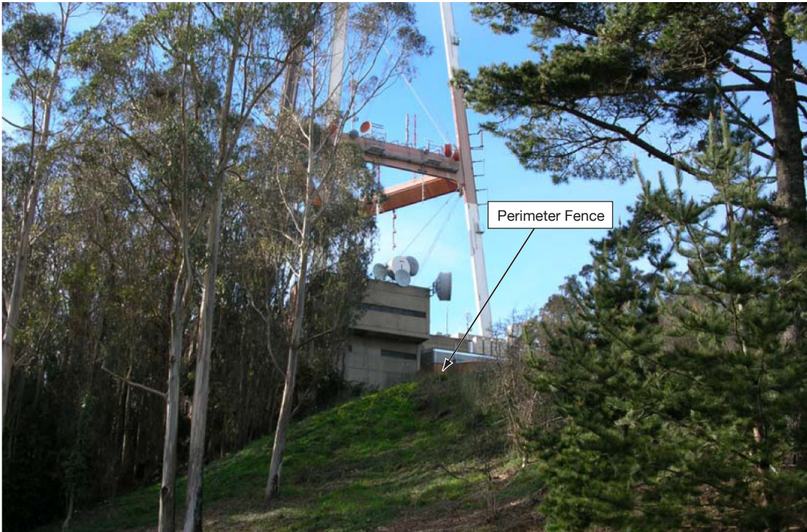
Base of Sutro Tower and Transmission Building seen from near the end of Farview Court
