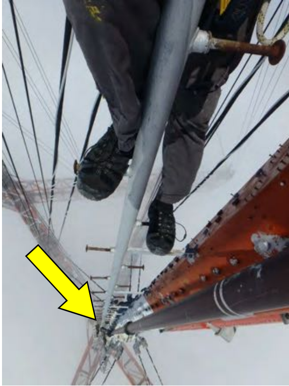
Missing Step Bolt Near Base at Climbing Pole
