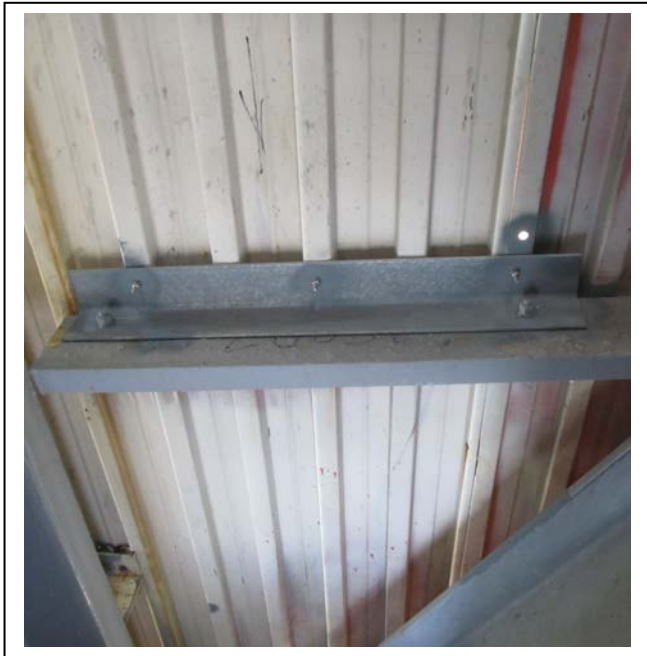
Photo No. 16 (After)
