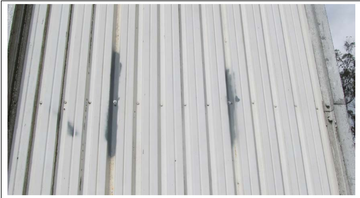
Photo No. 15 (After)
