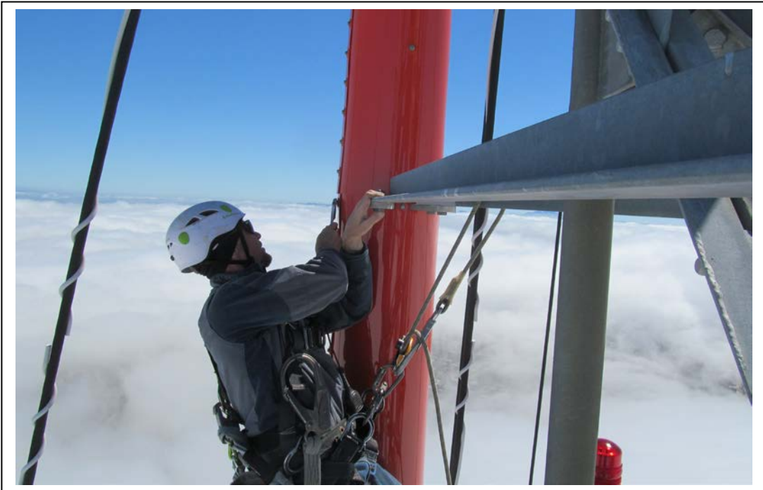
Photo No. 4 (After)
