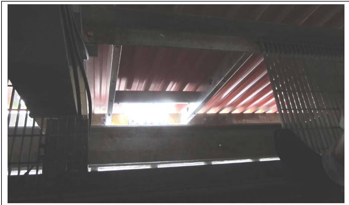
Photo No. 10 (After)
