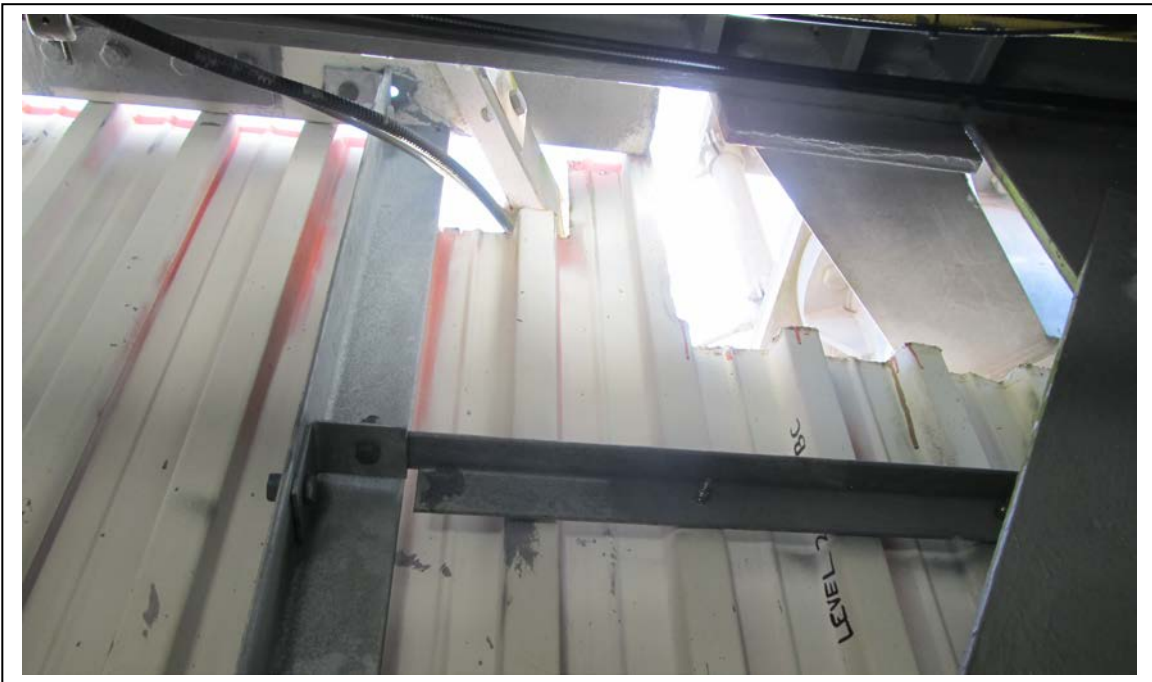
Photo No. 8 (After)
