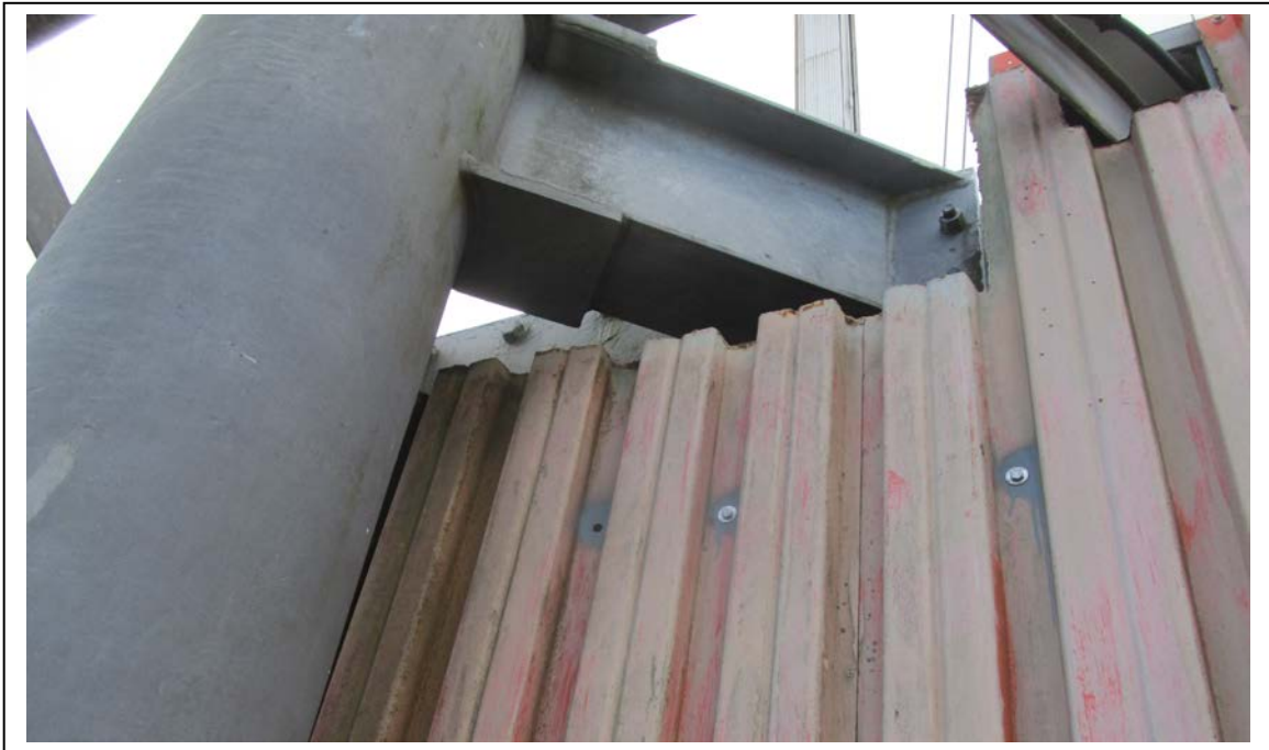
Photo No. 12 (After)
