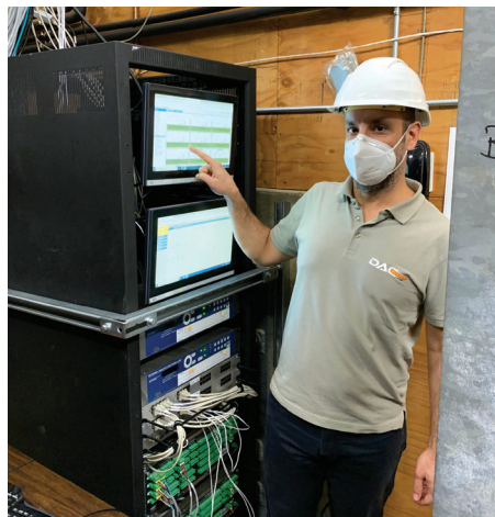
Maurizio Santovito in one of the antenna monitoring control rooms
